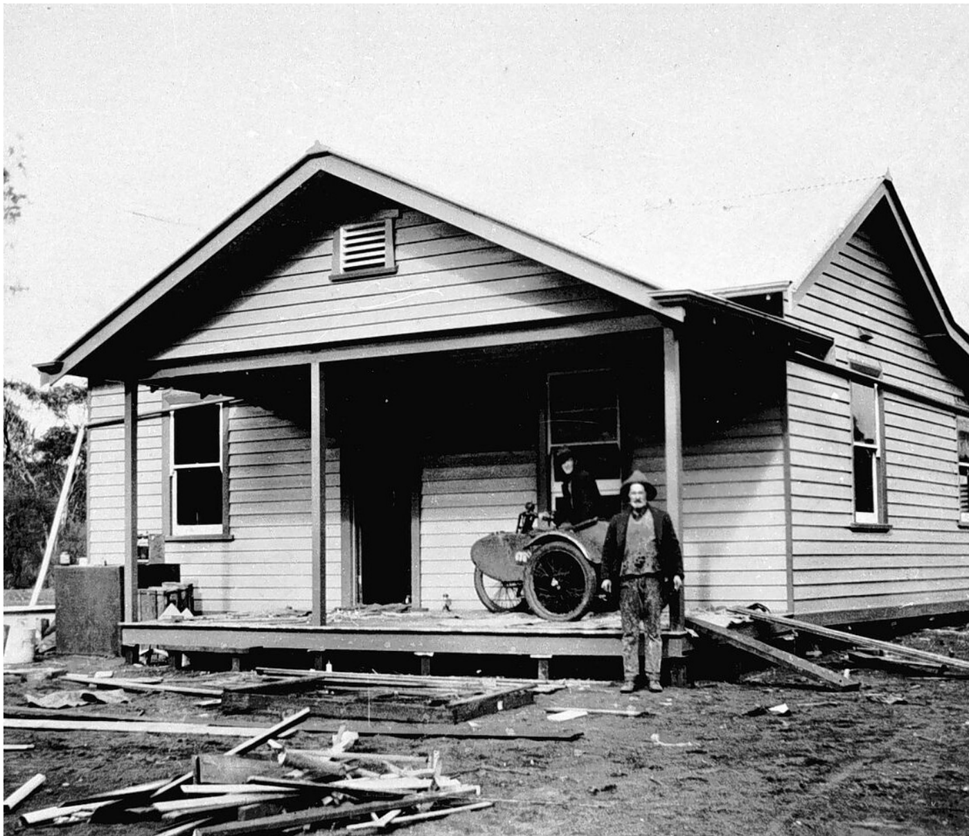
A PIONEERING FAMILY HOME UNDER CONSTRUCTION AT WERRIMULL.
